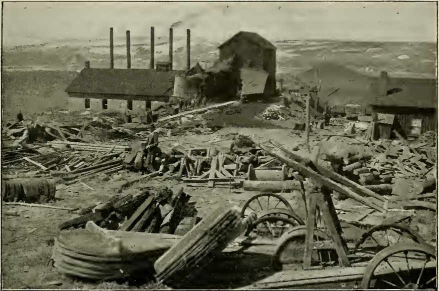
ENGINE AND BOILER HOUSE IN FRONT OF MAN AND CAR DRIFT.
